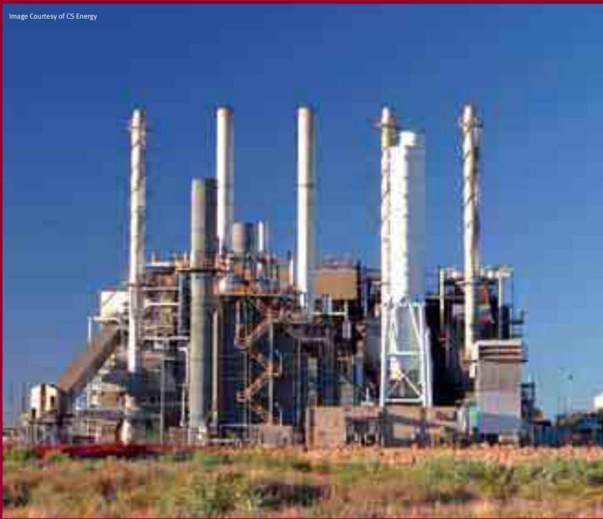
Mica Creek Power Station
