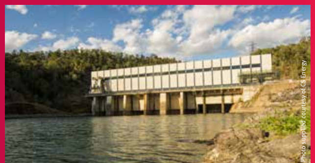
Wivenhoe Power Station
